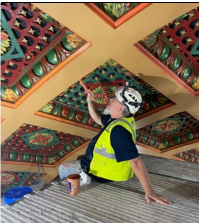
A painter painstakingly restores ceiling carvings to their original glory atop scaffolding erected inside the Florida Theatre.
