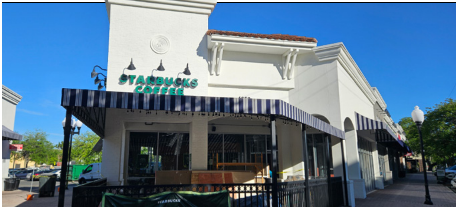
The Starbucks on Margaret Street closed March 15 for renovations.
