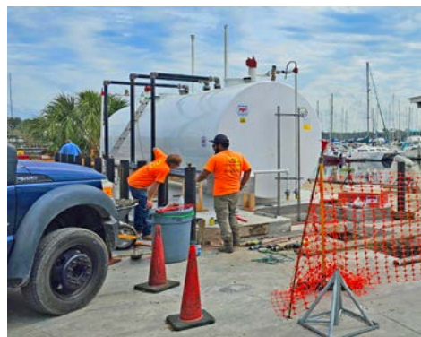
Crews working to install the new fuel tanks Windward Marina Group has brought to the marina.
