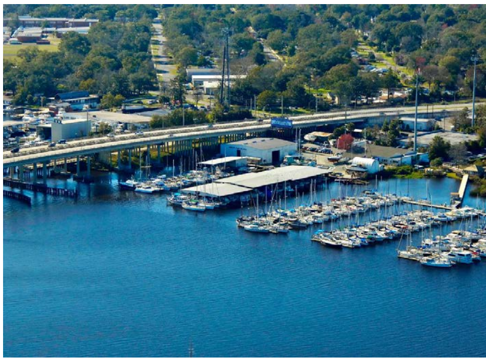
This image illustrates the property at Sadler Point (Left, under the bridge at US 17 or Roosevelt Blvd), adjoining to the former Ortega River Marina, which are both now part of the Windward Marina Group's acquisition and merger of the two marinas.
